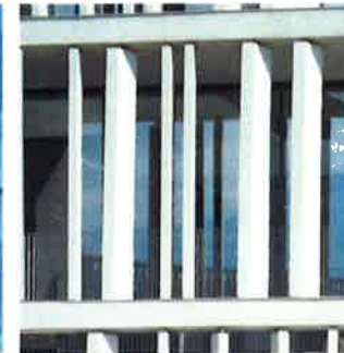
11. GLASS REINFORCED CONCRETE LOUVRES
