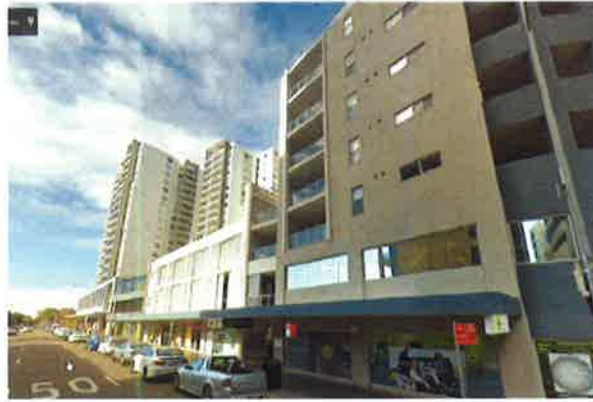
EXISTING MULTI-RESIDENTIAL BLDG 103 GEORGE STREET
