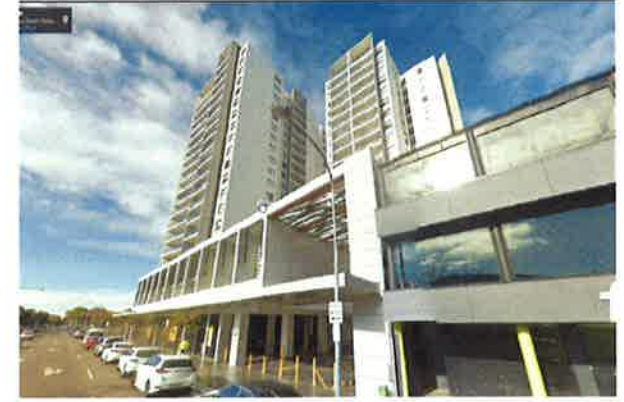
EXISTING MULTI-RESIDENTIAL BLDG 109-113 GEORGE STREET
